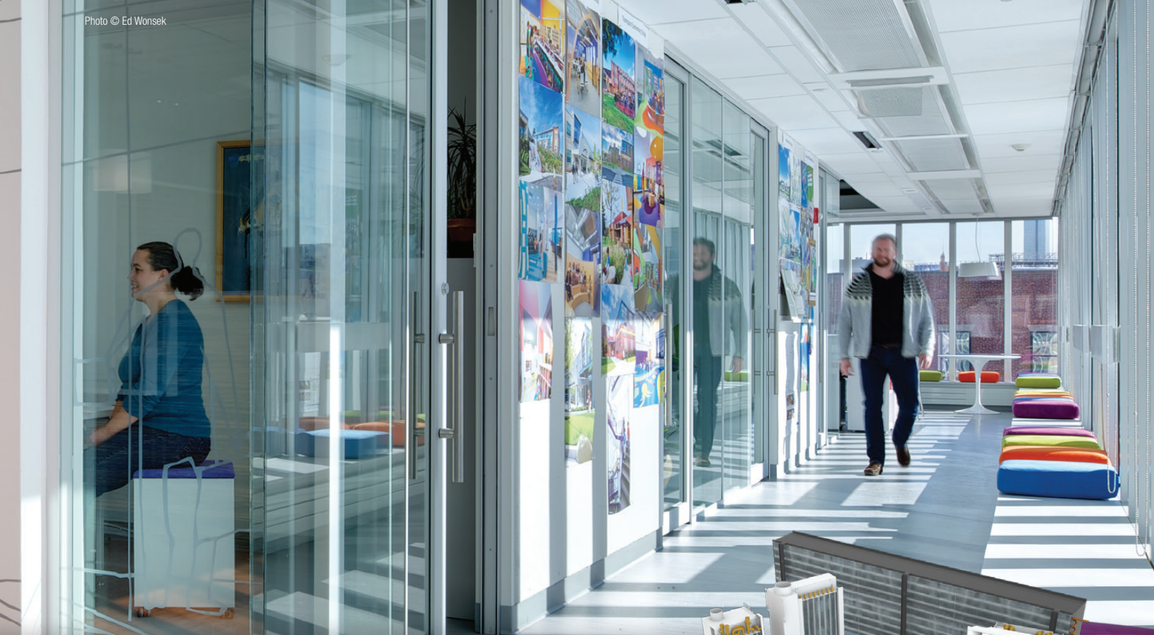
Above: Chilled Beams
